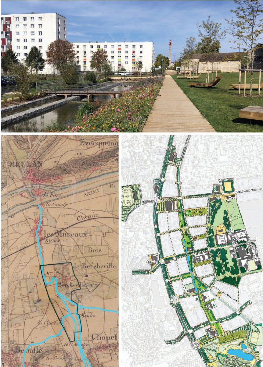
FIGURE 16.3 Les Mureaux . Image on the left. To the south of the village of Les Mureaux, the watercourse of Orgeval (highlighted in blue) which used to meander in the “open air” at the foot of the slopes of the Bois de Bécheville was made into a culvert during the construction of the large housing complex, “erasing” the geography of the site – extract from the map of the Etat Major, 1866 ( https://remonterletemps.ign.fr ). At the foot of the hill, extending out from the parc du Sautour, the watercourse was opened up again, creating a linear park that connects the districts and their facilities. On the slope of the hillside, the “garden avenues” connect the Bois de Bécheville to the linear park, supporting gardening and leisure activities in the neighborhood. Image on the right. The linear park and the Bécheville garden avenue. © germe&JAM.
